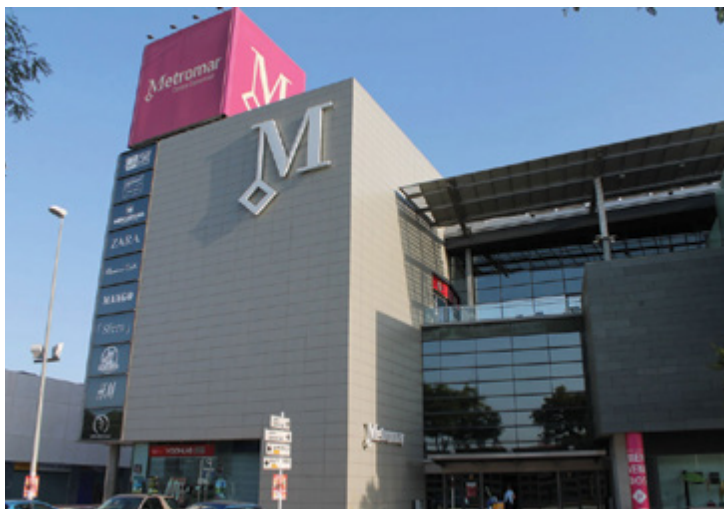
Metromar Shopping Center, Seville
